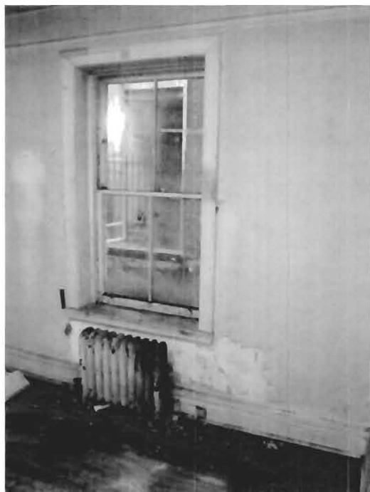
Subject: Living room of a vacant unit. (Water damage, stained floors, poor waterproofing around window, & uneven floor)
