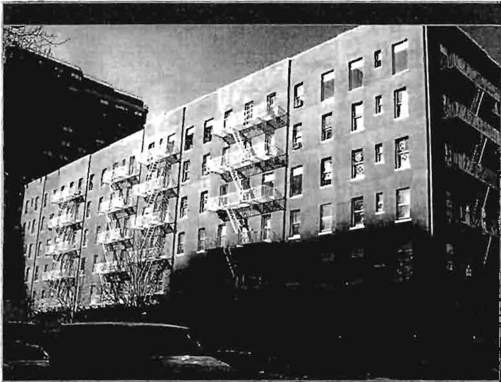
View of the subject property looking southwest across York Avenue.
