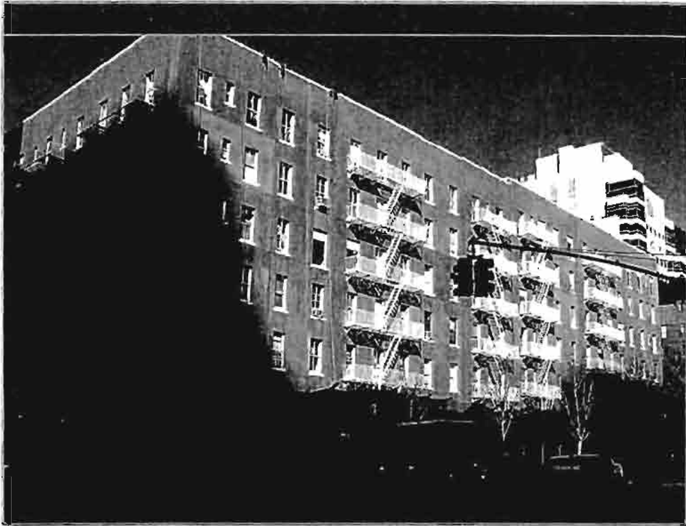
View of the subject property looking northwest across York Avenue.
