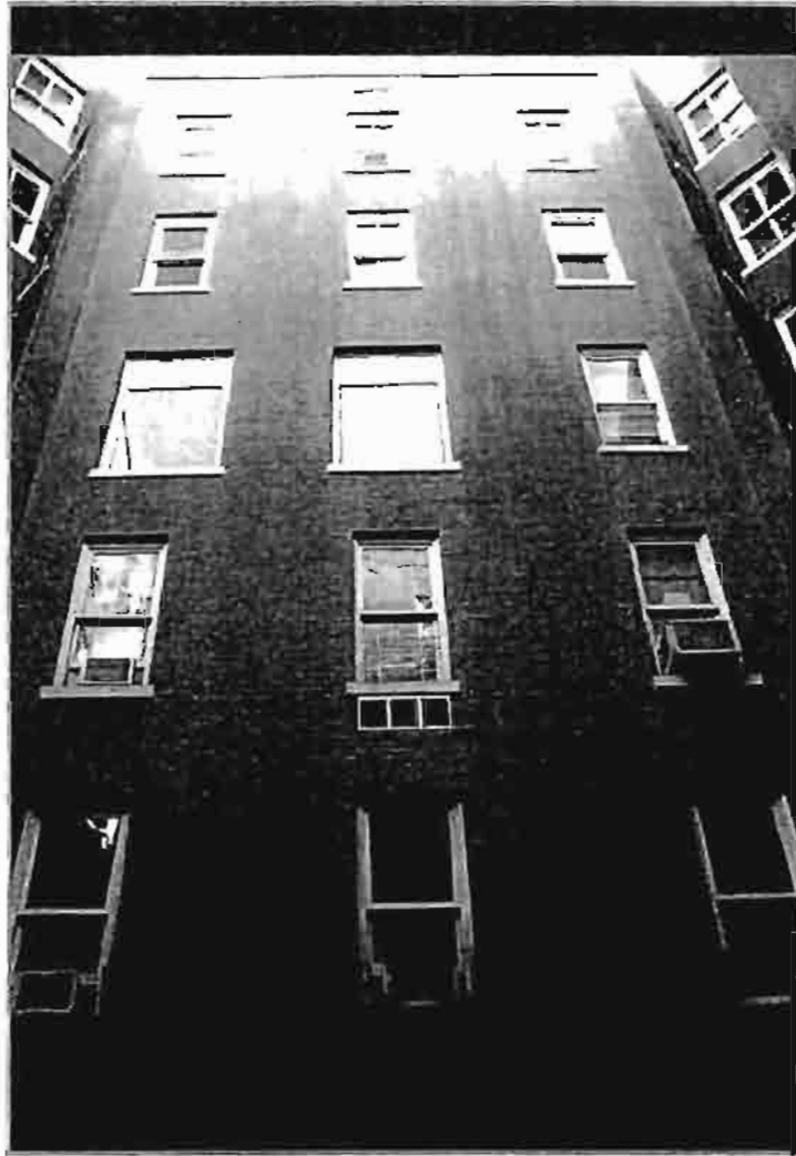
View of exterior façade facing courtyard.
