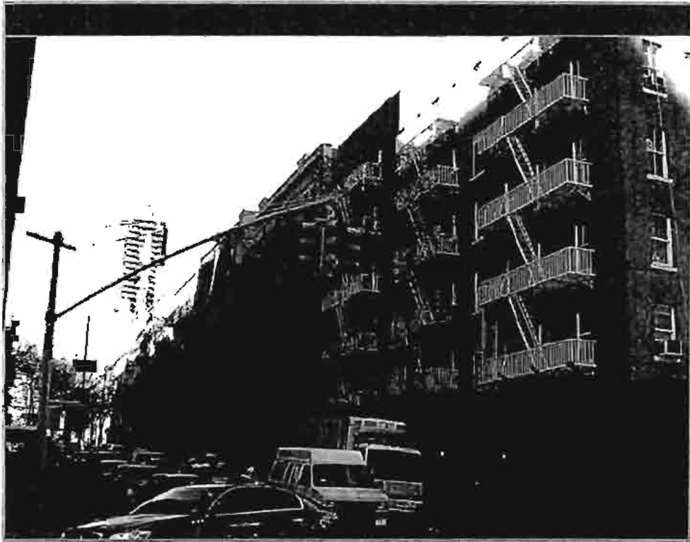
View of the subject and adjacent buildings from East 64 th Street.
