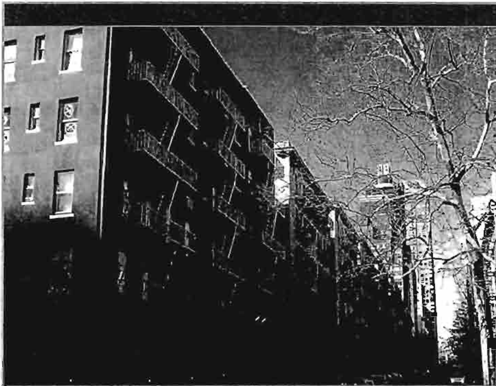
View of the subject and adjacent buildings from East 65 th Street.
