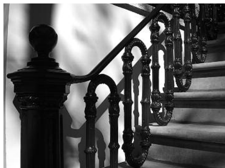
Restored railings at No. 129 East 70th Street
