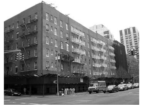
York Avenue façade of First Avenue Estate, conditions in December 2007.
