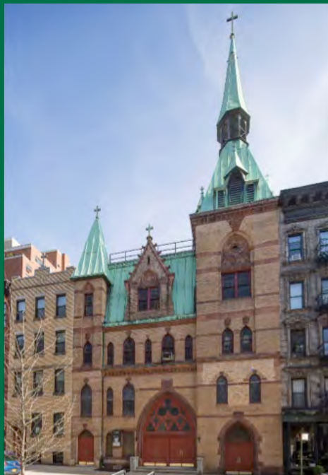
St. Elizabeth of Hungary at 211 East 83rd Street, constructed in 1893, is one of the many extant buildings which tell the story of Yorkville's immigrant past.
