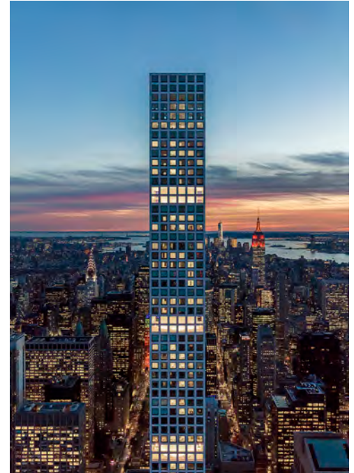
432 Park Avenue at night. Each pair of illuminated floors is mainly empty space.
