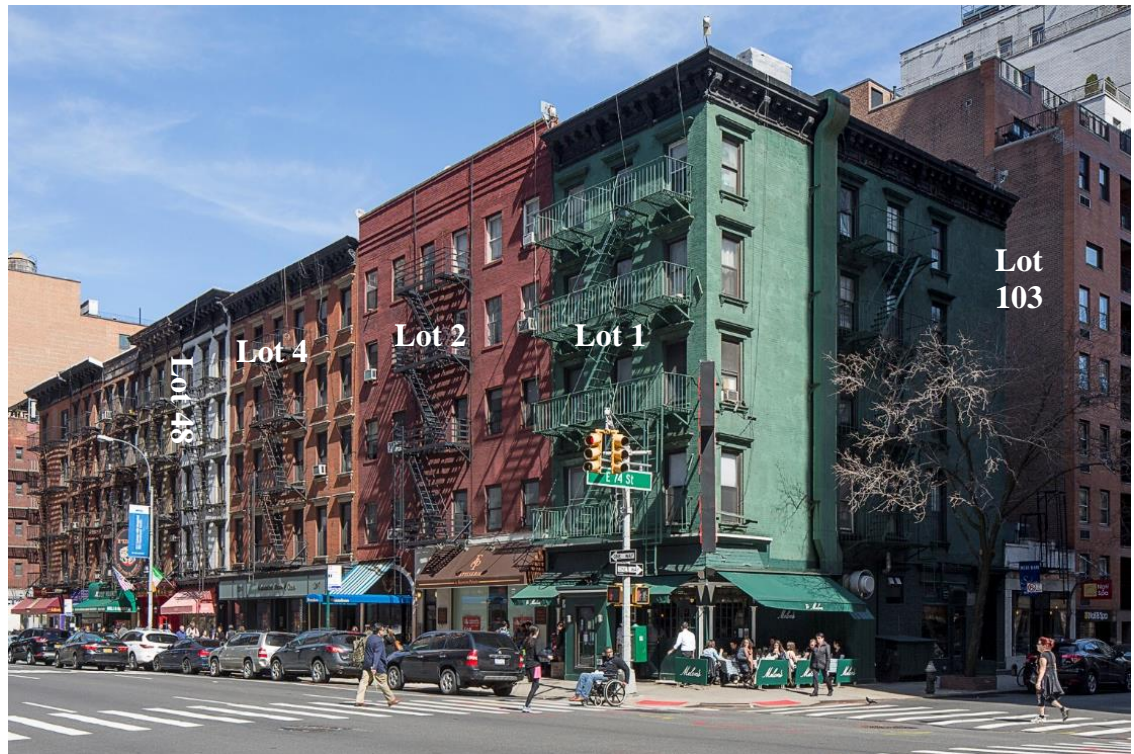
Preconstruction photograph of the development site. The “Lot 4” buildings have been demolished and the new building will be located here. Other buildings to stay on the zoning lot are numbered with their lot number.
