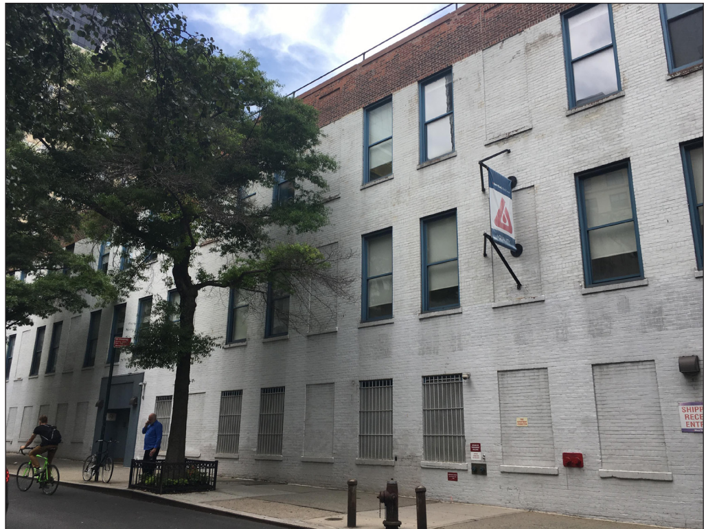
View of Development Site looking northwest on East 66th Street 4
