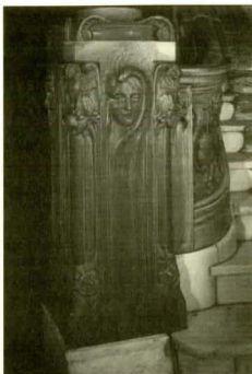
Detail of the terra cotta newel post on the staircase inside the New Amsterdam Theater, 214 West 42nd Street. Photo: Friends of Terra Cotta
