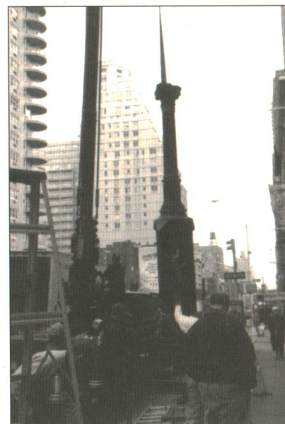
Next to be hoisted away is the stanchion.
