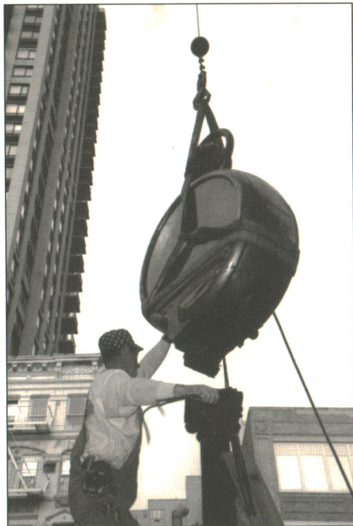
The clock's head is lifted right off its cast-iron stanchion.
