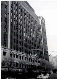
At the Westbury Hotel, 828 - 850 Madison Avenue, work will include a major face lift. Cornices and limestone balconettes will be restored, and through-the-wall air conditioner cuts will be patched with matching brick.
