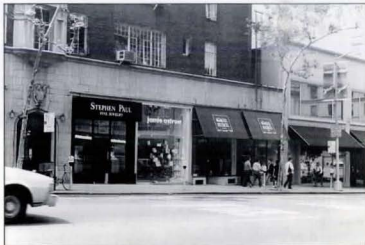
874 - 876 Madison Avenue. The Stephen Paul and Jamie Ostrow stores are in violation. Historic storefront fabric (evident in the Alain Mikli store, i.e., tri-partite division, entry vestibule, and cast concrete bulkhead) have been removed. This would be a Type A violation.
