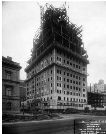
720 Park Ave under construction
