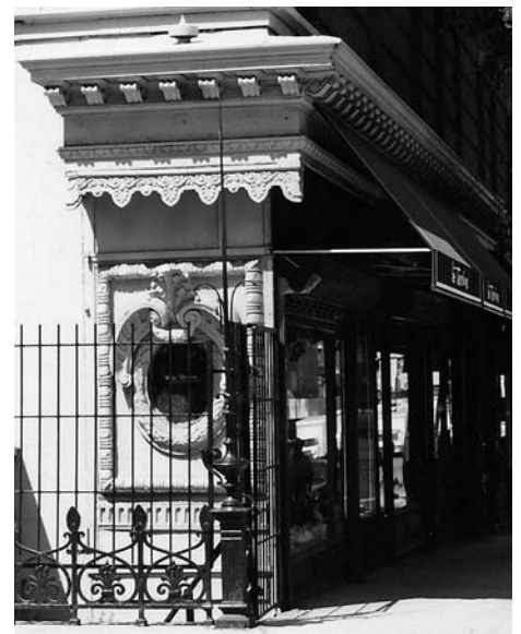
133-137 East 73rd Street showing saved cartouche
