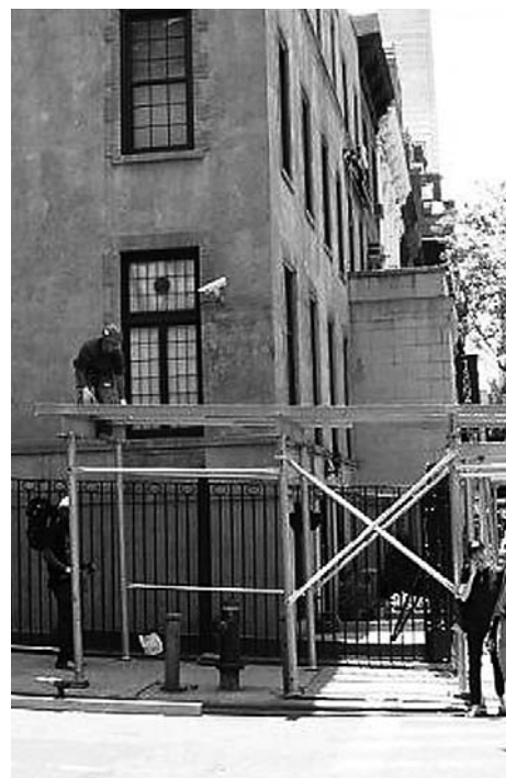
Workers erecting scaffolding outside the Kean Residence, July 2008
