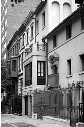
East 63rd Street between Lexington and Third Avenues
