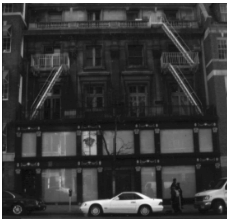
THE SOON-TO-BE-REMOVED CAST IRON STOREFRONT REMINISCENT OF THE ORIGINAL 1933 ALTERATION.
